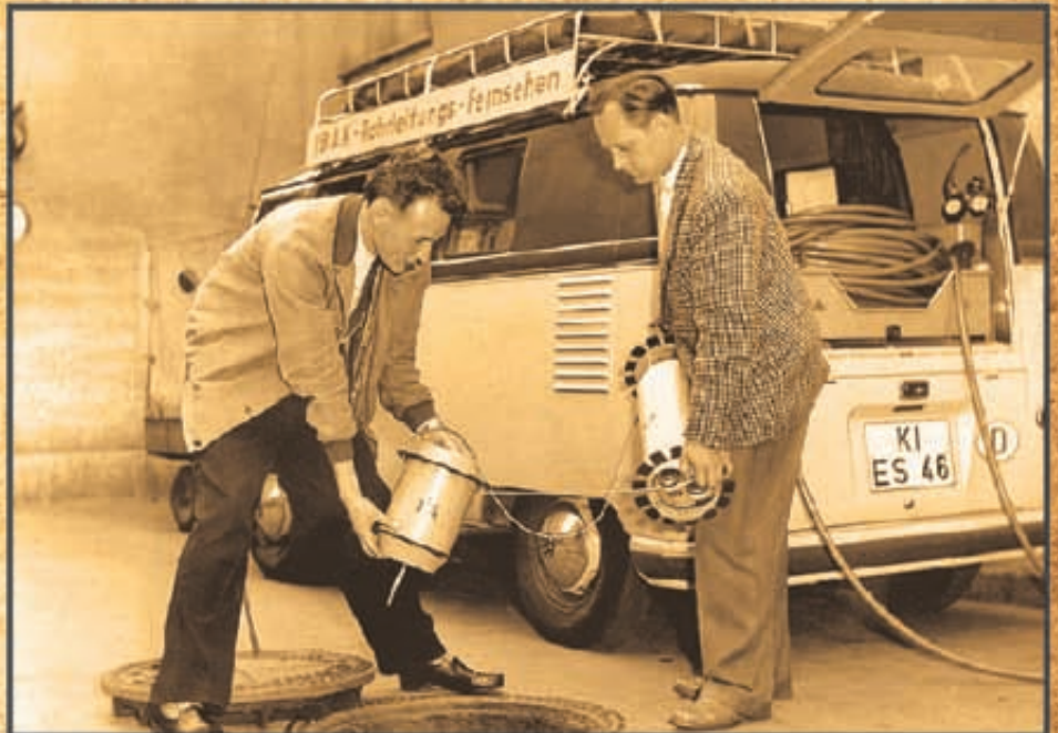
This amazing new technology is lowered into a manhole - where it records pictures of the underground world!
