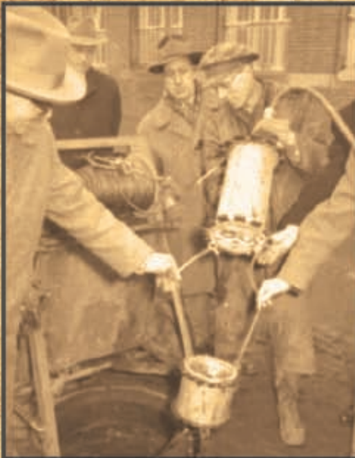
Workers lower the first camera of its kind into the manhole.
